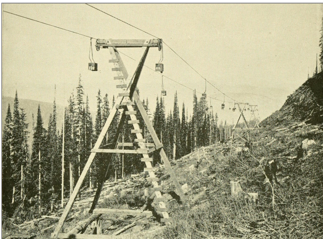
"Towers on ropeway at Hall Mines, Nelson, B.C." The aerial tramway carried Silver King ore down to the smelter.
